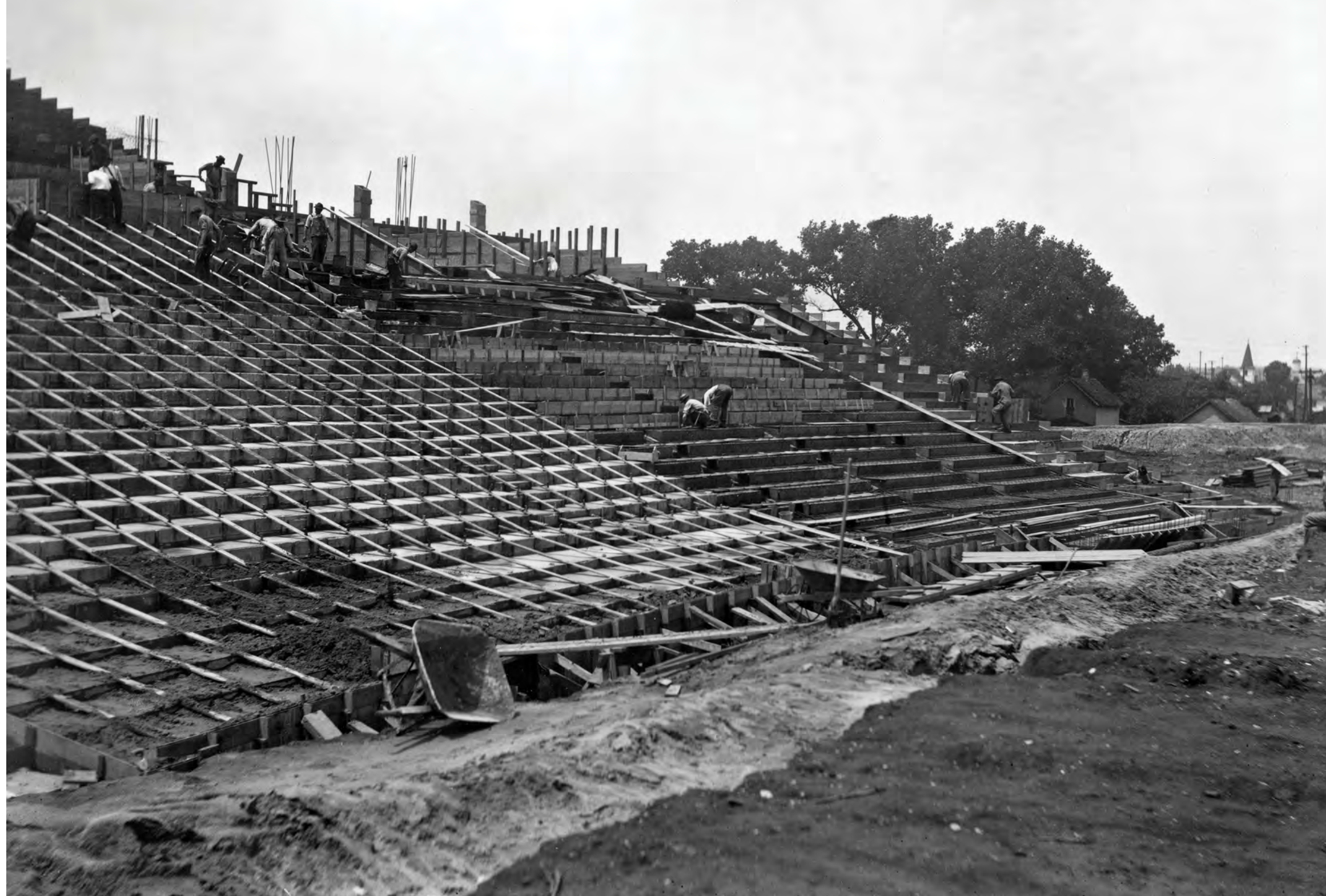
Memorial Stadium under construction, 1923. HISTORY NEBRASKA, RG2758-21-8
