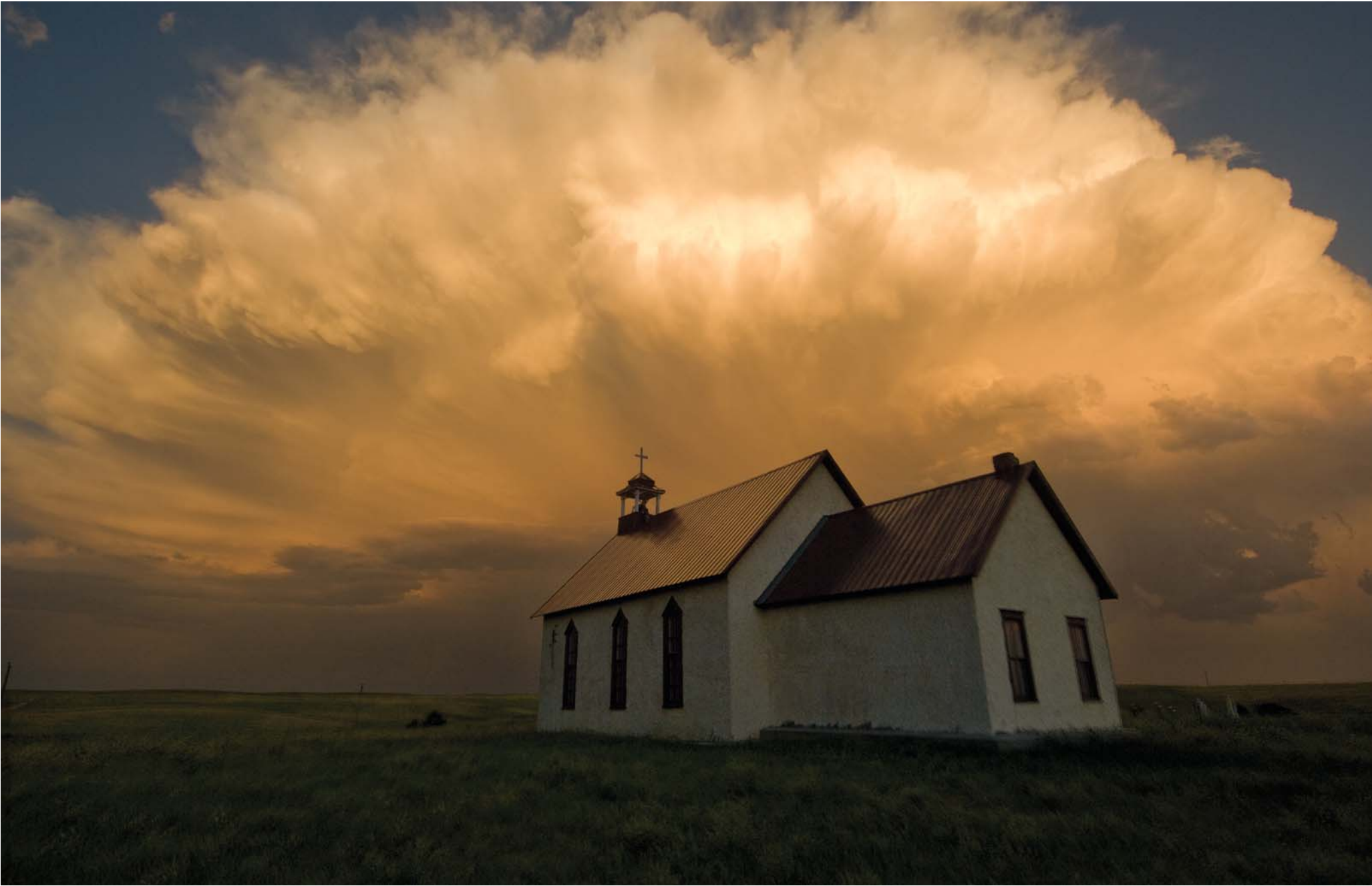
Montrose Church, a landmark on the grasslands of northwestern Nebraska, was built in 1887 and is still in use today.
